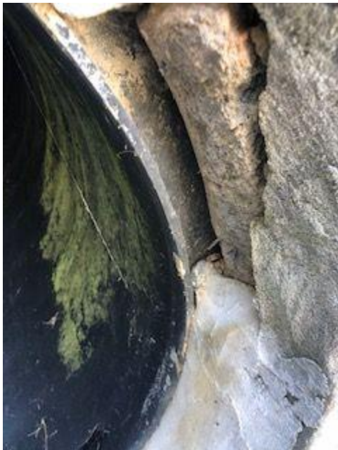
Photograph No. 3 – Close up photograph of separation of pipe and concrete at EW-2.
